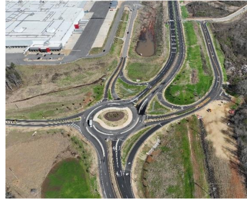
This is the completed “turbo” roundabout adjacent to the new Smucker’s plant in west Jefferson County. It was a part of a widening of Old Tuscaloosa Hwy., which serves one of our industrial parks.
